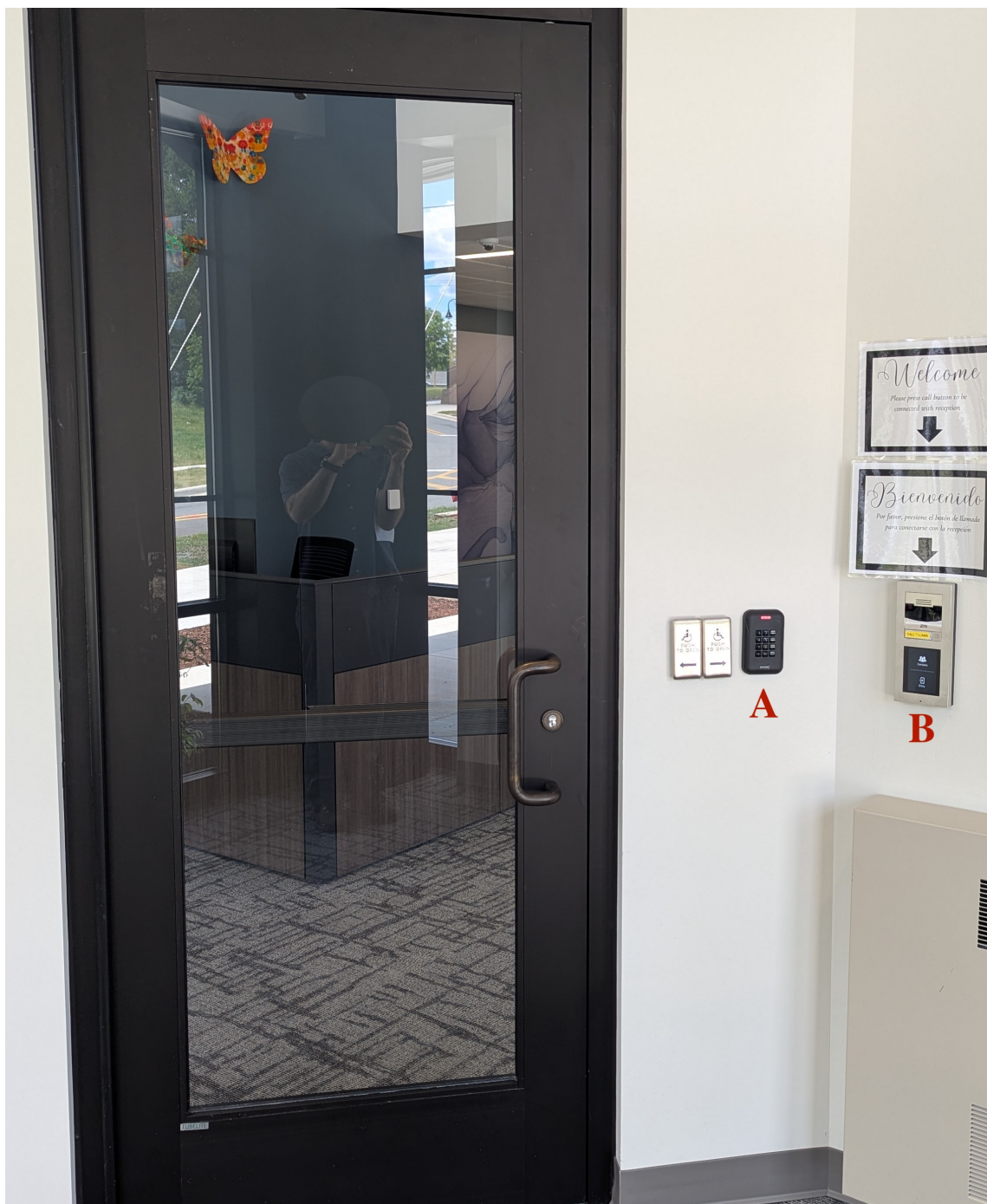
Figure 2: VFPC main entrance, inner door. (A) Electronic Lock, (B) reception page.
