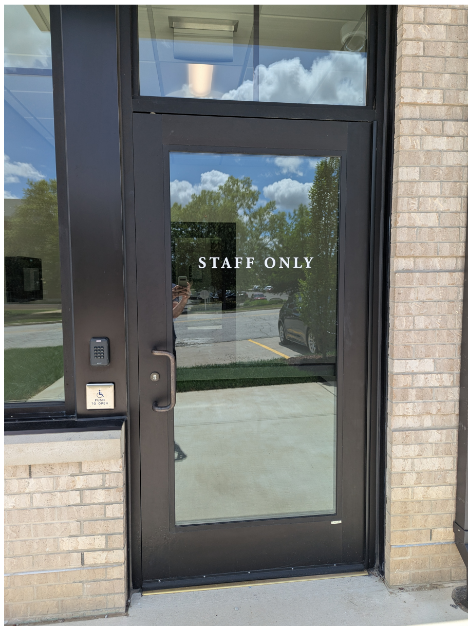
Figure 4: VFPC staff entrance, south.
