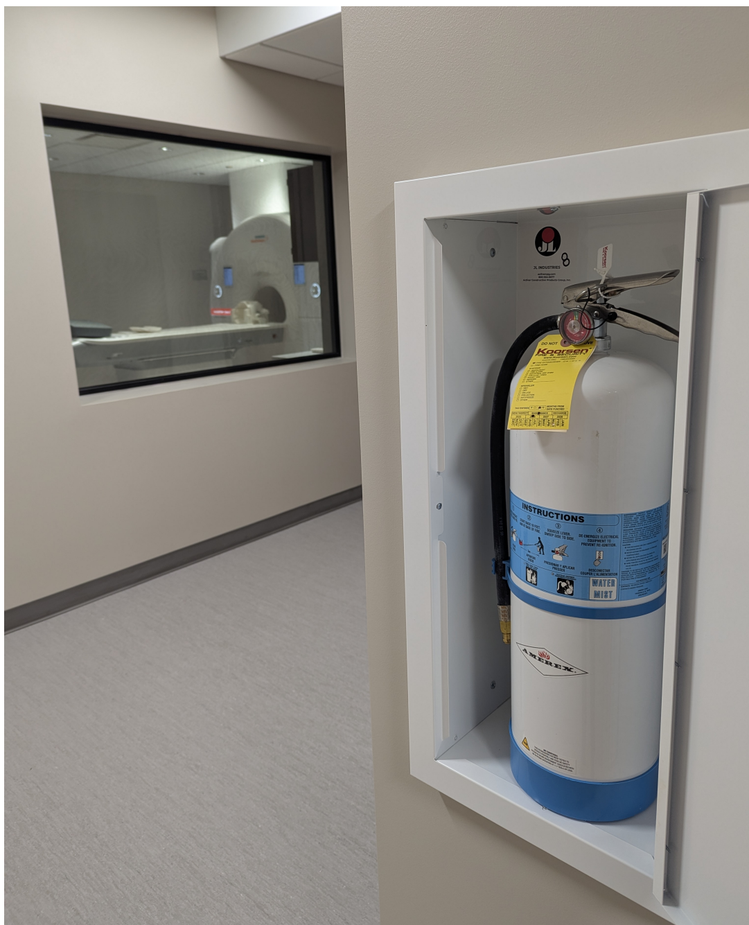
Figure 4: Zone 3 (B15) MR-compatible fire extinguisher.
